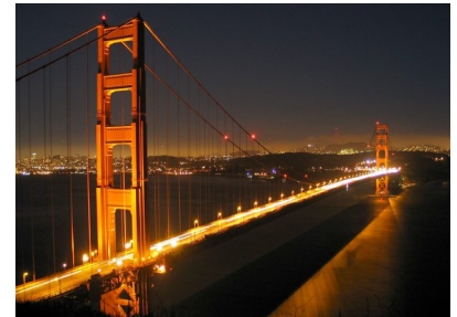
o / The Golden Gate Bridge's roadway is held up by the tension in the vertical cables.
